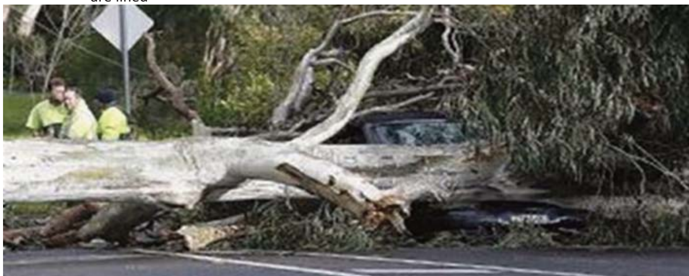
Eltham Gateways Main Road blocked in normal storm conditions (DV Leader 6 September 2012)
